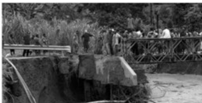
Flooding in February 2005 led to the disruption of the Lae-Madang Highway, a main transport route in PNG.
