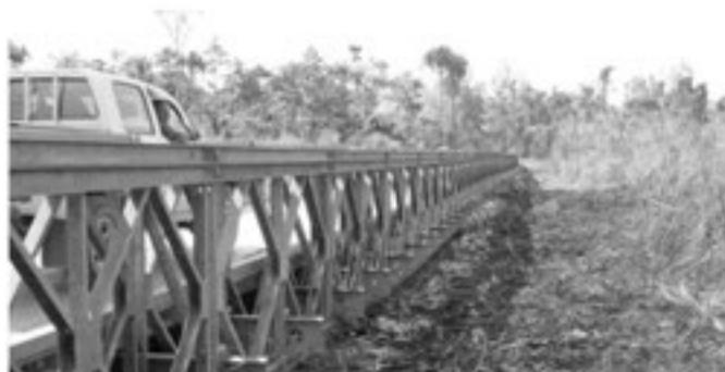
Floods can transport a huge amount of sediments into oceans and onto reefs. At this bridge in PNG the whole river channel was filled up with sediment over a distance of 20 km. The river channel disappeared altogether within 3 - 5 years. This bridge worth a million kina became redundant and was dismantled.
