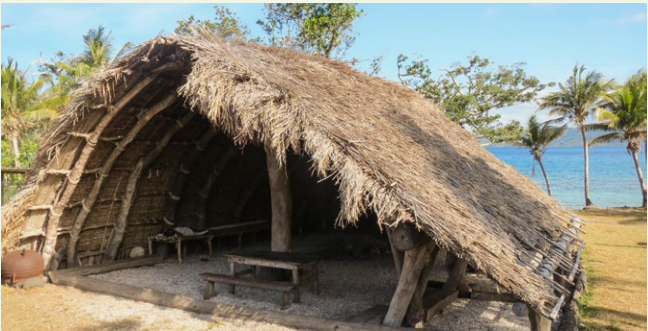
Figure 6: The nakamal in Taloa, made from local materials, appears solid and safe. It provided shelter mainly to young men from the community and suffered only minor damage during the cyclone.
