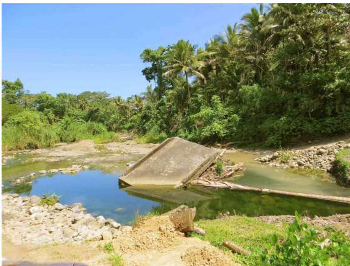
(Collapsed bridge along main road in South Santo leading to Wailapa)
