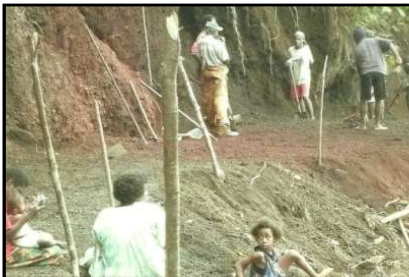
(Road works completed with hand-held tools in South Epi- 2013)
