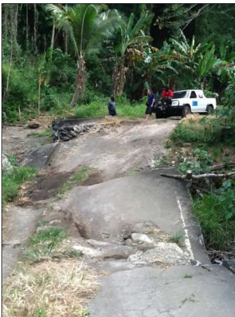
Figure 1: The collapsed bridge in the Epi Project site.
