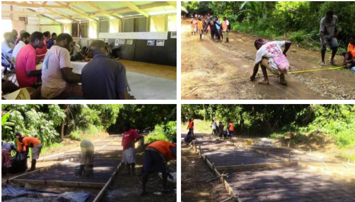
Figure 9 Illustration of the work conducted by PWD to construct concrete tracks and train local labour (Ian Lercet / PWD 2013)
