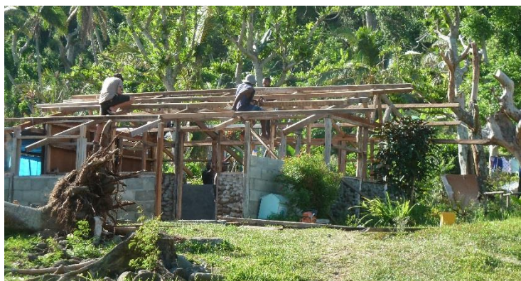
Rebuilding houses after Cyclone Pam in Dillons Bay, Erromango.
