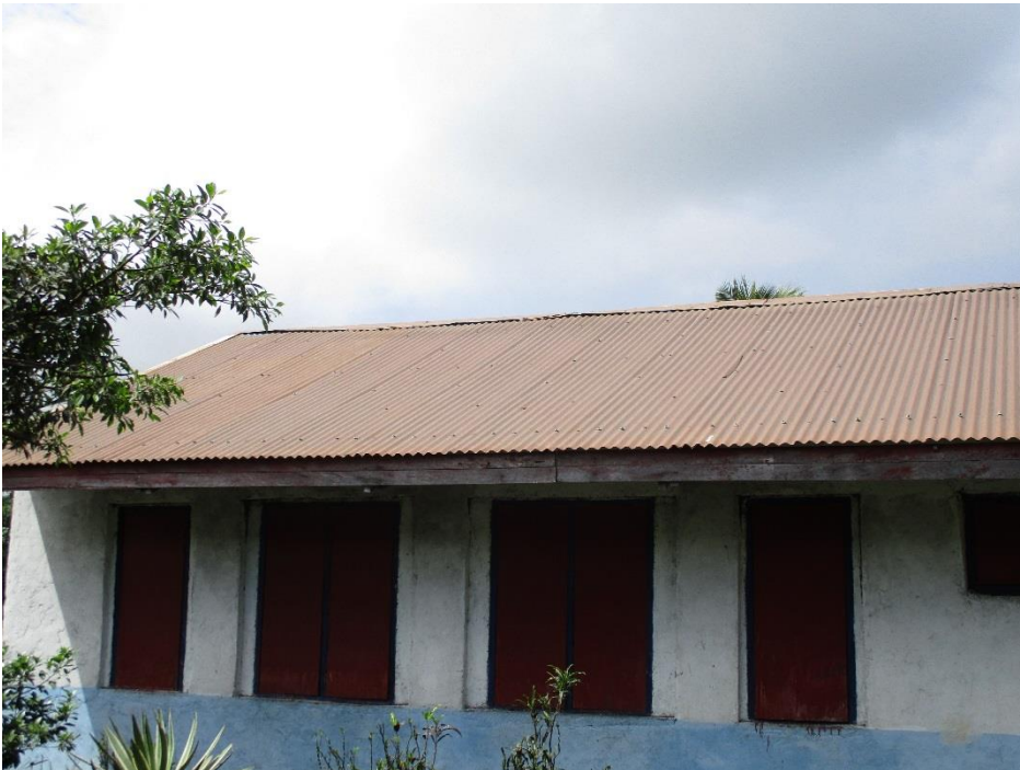
Figure 1: Suitable North Facing Roof for PV System at Divain School
