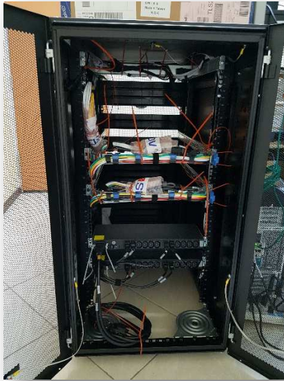
Cabinet during the installation
