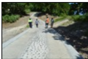
EPI ROAD NEARING COMPLETION
