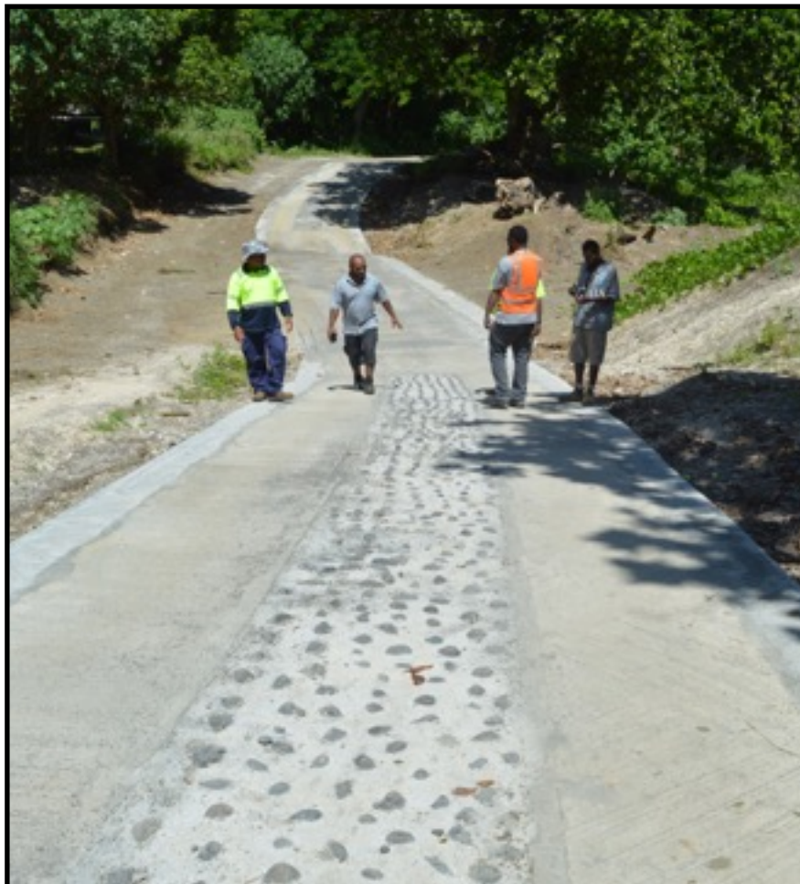
Malvasi Creek Drift Crossing
