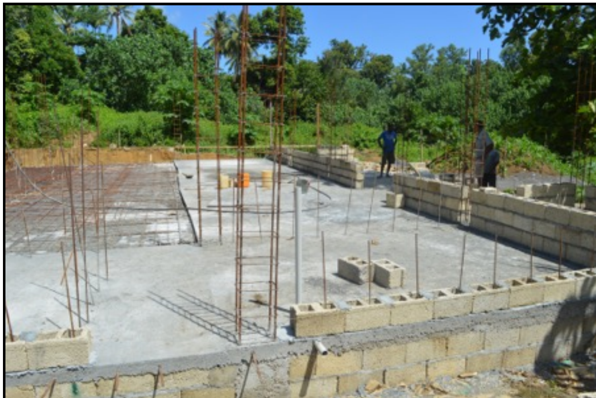
Foundation of Vermaul Area Council building in Rovoliu, Epi.
