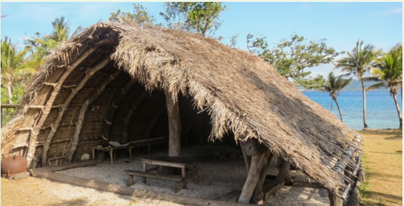
Figure 6: The nakamal in Taloa, made from local materials, appears solid and safe. It provided shelter mainly to young men from the community and suffered only minor damage during the cyclone.
