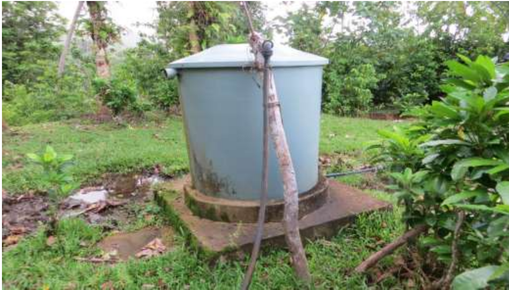
1,000 litres of storage poly tank in Savat Village.
