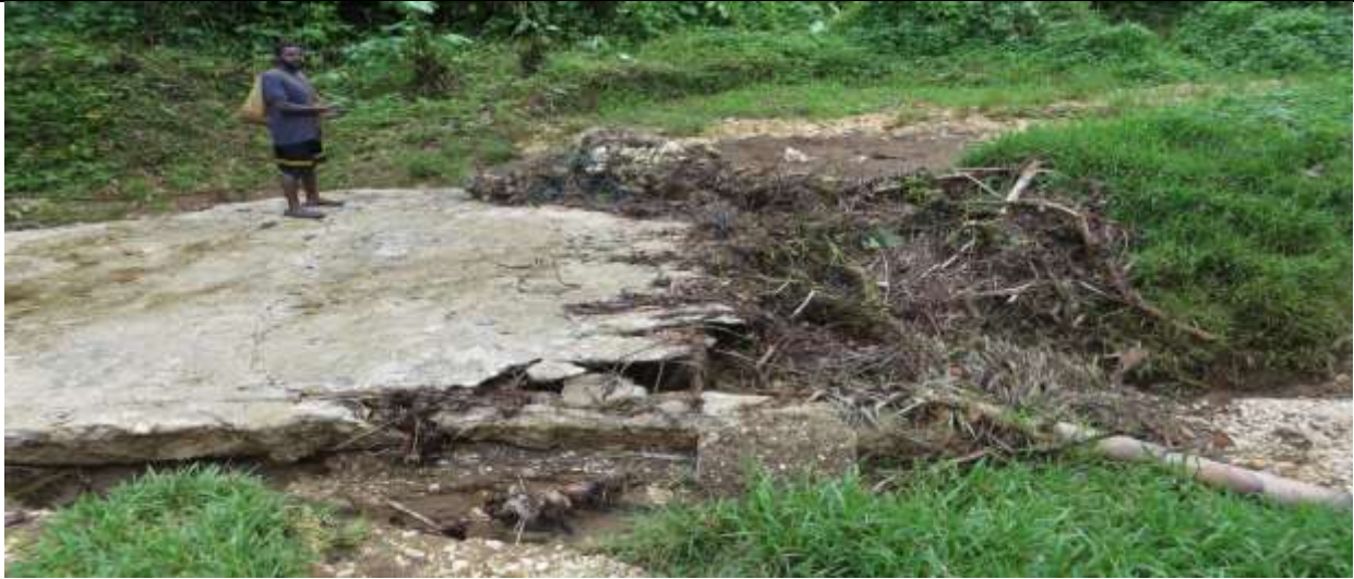
Damaged Concrete Crossing at Portugal-CP2
