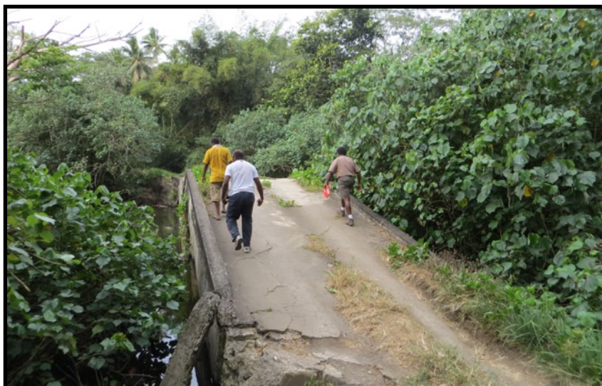
(Collapsed bridge near Yervali School is no longer accessible to vehicles)
